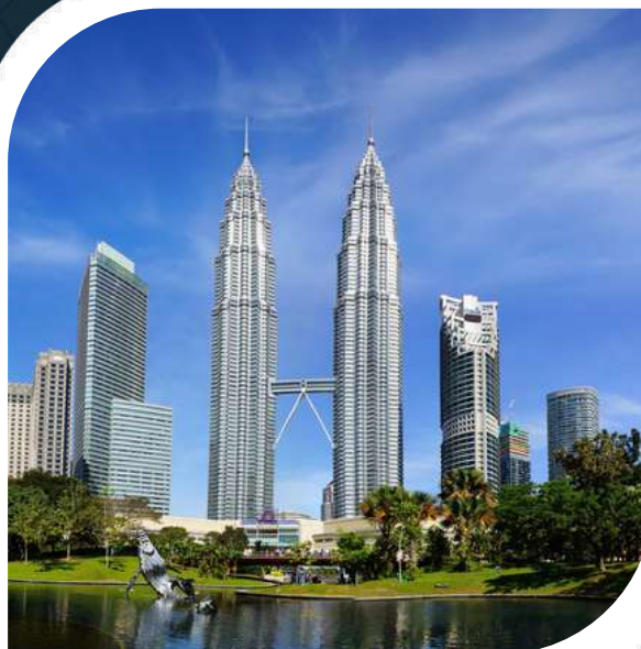
Petronas Twin Towers
