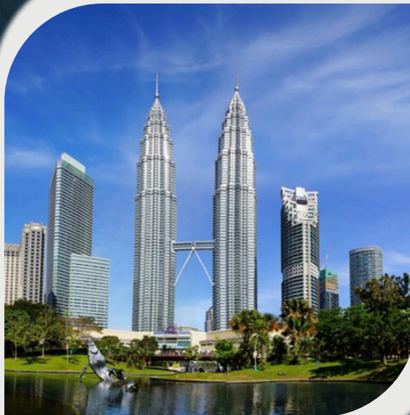
Petronas Twin Towers
